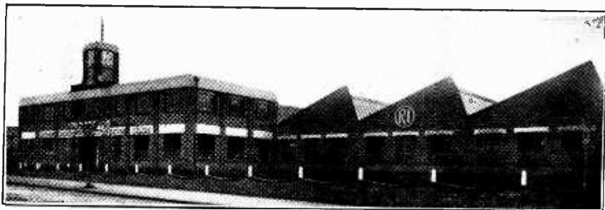
BUSIER AND BUSIER. This view of the three new bays (on right) which have just been added to the Croydon factory of Radio Instruments Limited, tells its own story. Accommodation is provided for a further 250 employees, most of whom are busy on R.I. transformer construction.
